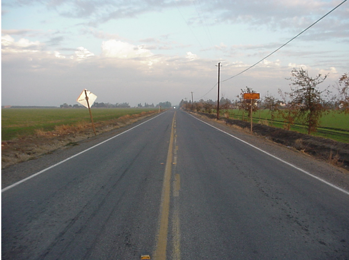
Figure 2 – County Road 29 east of County Road 99 (11' vehicle lanes, gravel shoulders)
