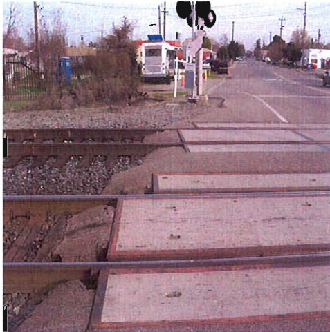
Location No. 3 - A Street
