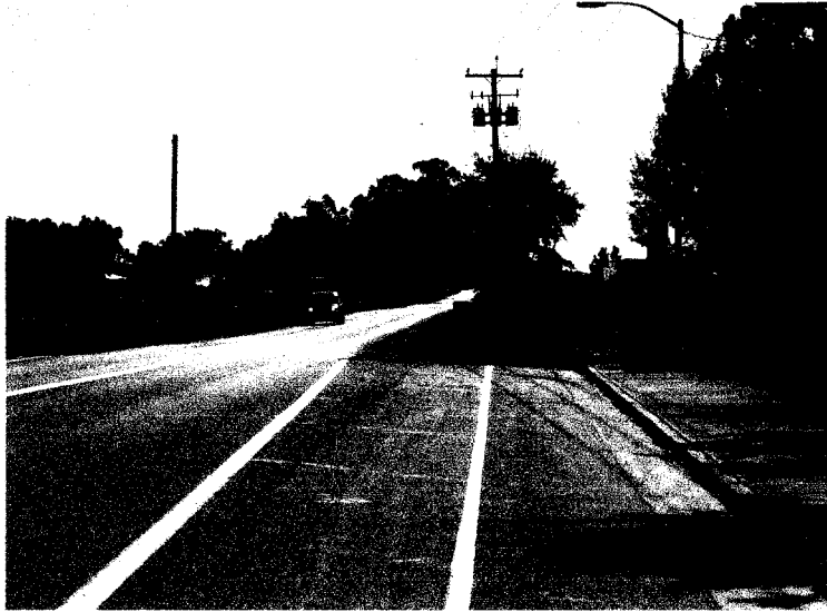
Looking south on Marengo Rd.
