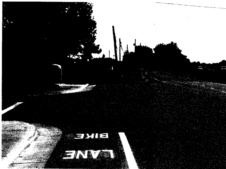
Looking south on East Stockton Blvd. past Adare Way.
