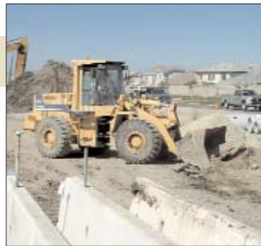
Caltrans begins construction on one of 50 local projects.
