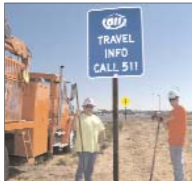
Caltrans employees install the 511 road signs.
