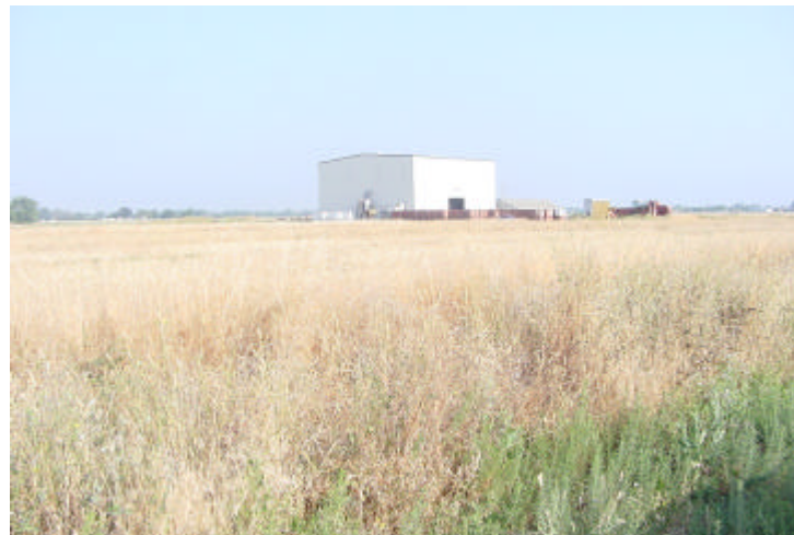
5 - Nor-Cal Rice processing plant, West of County Road 101
