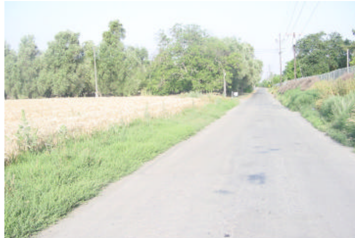
1 - Looking West on County Road 24A, West of old State Route 113
