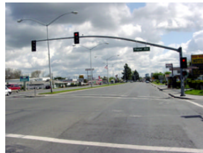
5 - West Capitol, looking East from Poplar
