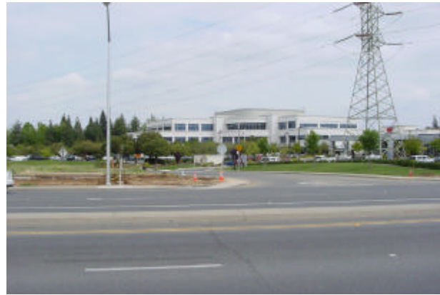
1 - County Traffic Court building & auto testing facility adjacent to transmission line corridor
