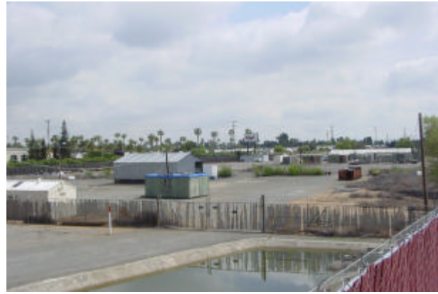
3 - Storage lot adjacent to substation
