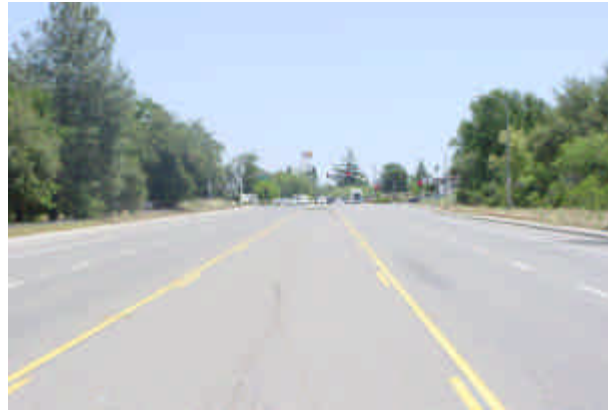
4 - Looking East on Granite Drive towards Sierra College Boulevard
