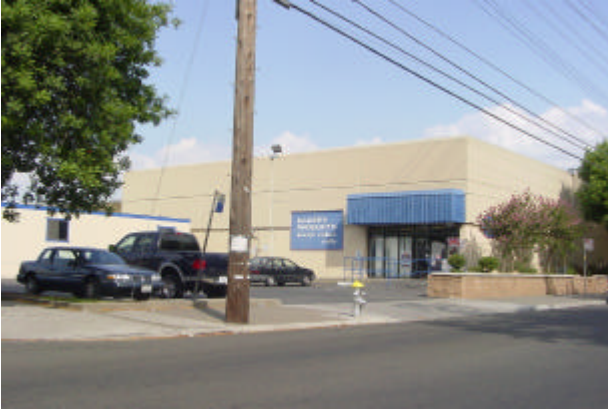
3 - Bakery outlet at corner of 6th & 33rd
