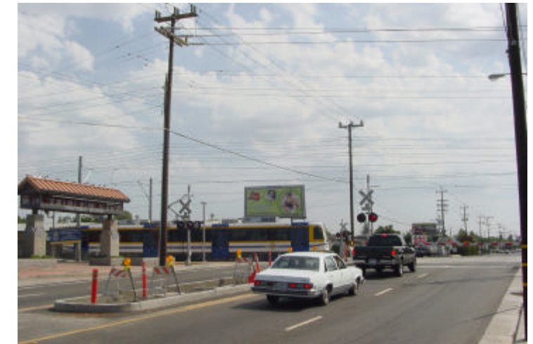
2 - New Light Rail Station at Fruitridge; adjacent to Union Pacific tracks
