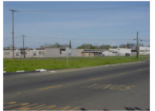
15 - Vista Nueva High School, looking North from North Ave
