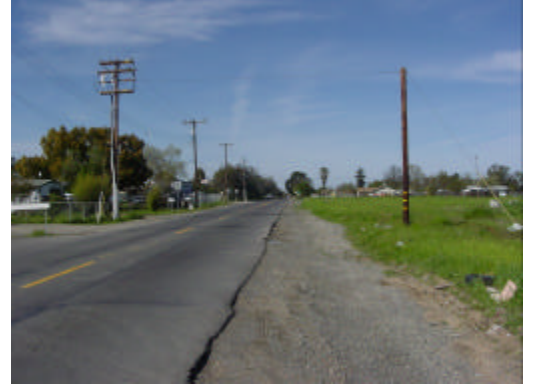
4 - North view along Raley from Vinci Ave intersection
