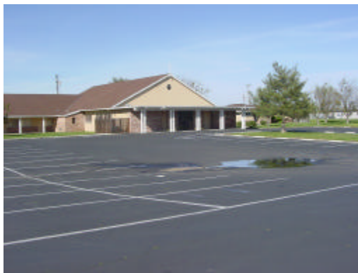
12 - Church on North Ave at Pinell St, looking Northeast
