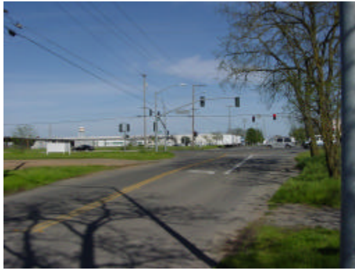
6 - Looking East on Main at Raley Blvd intersection
