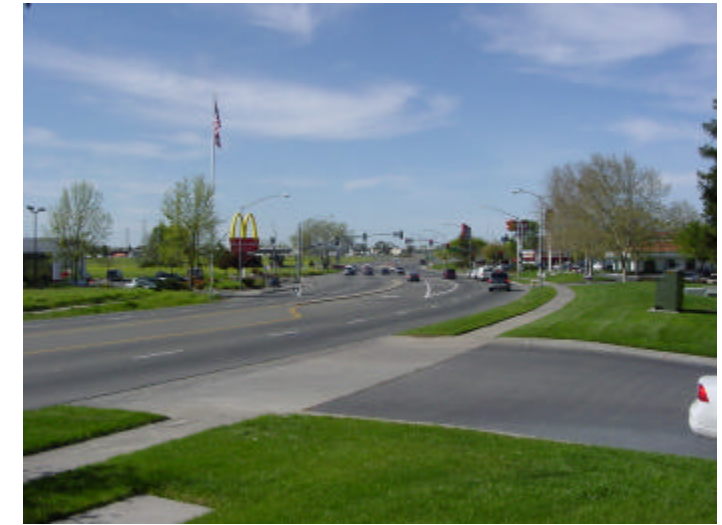
8 - North view of businesses along Northgate, South of I-80 interchange
