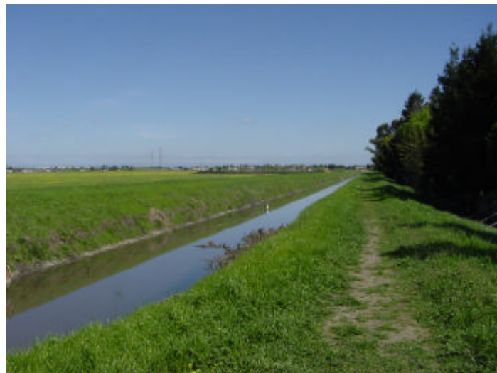
3 - Drainage channel just north of area of Single Family Homes
