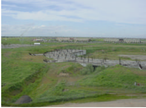
3 - View of lot north of Arena complex, facing Del Paso
