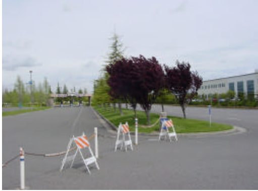
7 - Southeast Arena gate on left, Sports Pkwy businesses on right
