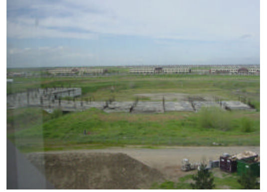
2 - Abandoned stadium foundation, North of Arco Arena
