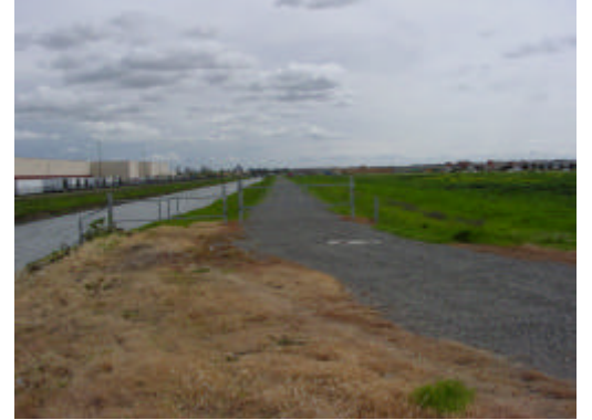
9 - Arena Blvd @ canal, looking South
