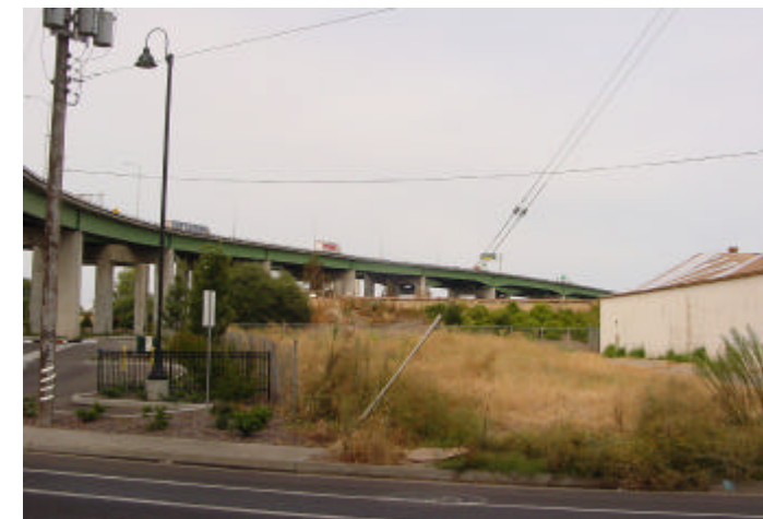
4 - Looking Southwest @ vacant lot behind Towe Ford Museum; freeway interchange in background
