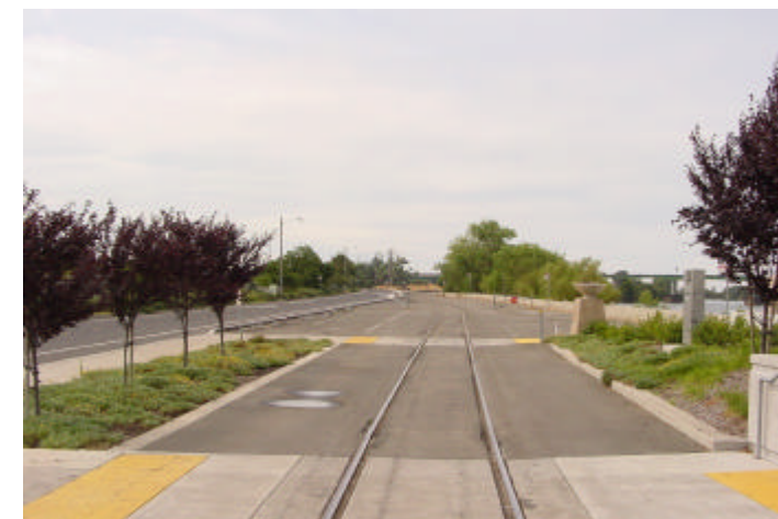
2 - Riverwalk, looking South; Sacramento River is off the right edge of photo
