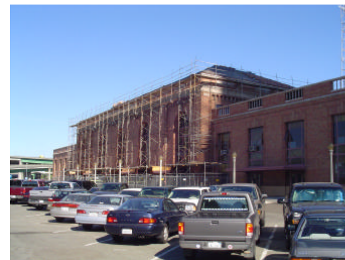
5 - Historic train depot on Southern edge of study area
