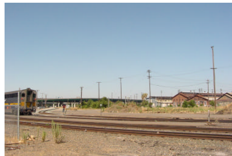
4 - Looking Northwest at locomotive works buildings; freeway in background
