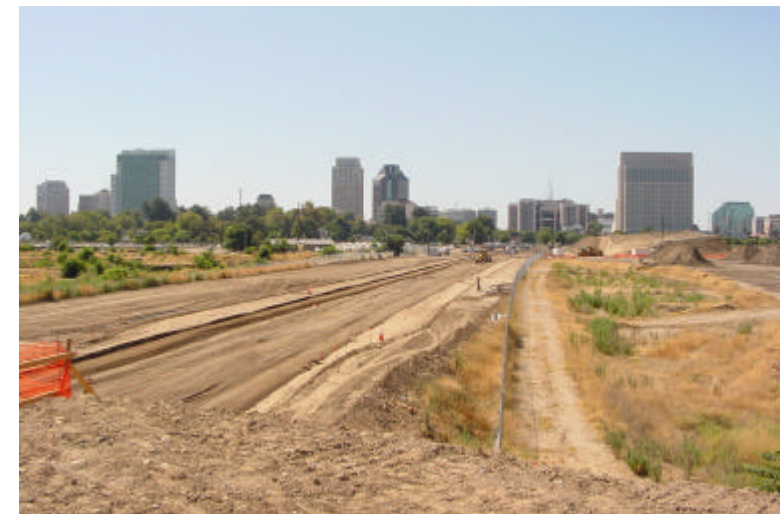
2 - Looking South along the construction of the 7th Street extension
