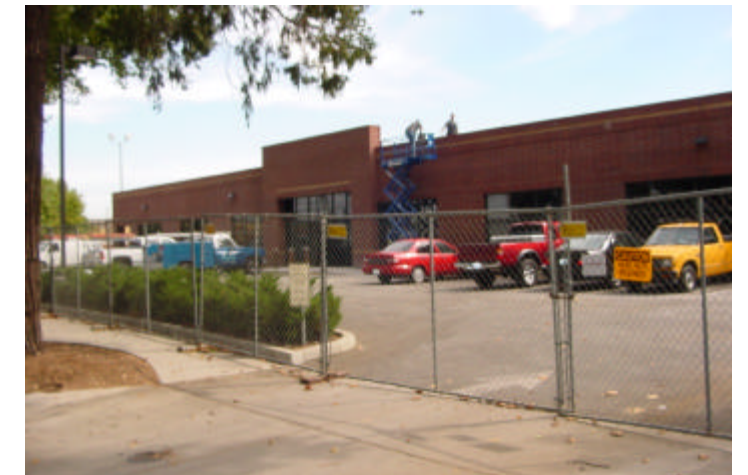
8 - New office construction
