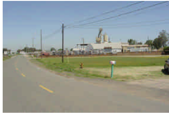
5 - Soil amendment product yard, looking Northeast along Crystal Way
