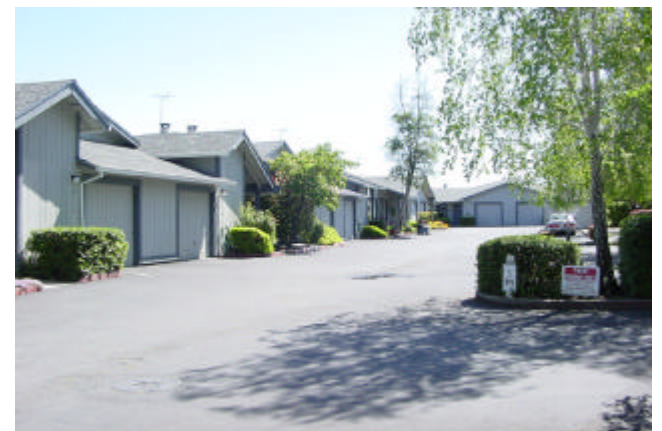
5 - Apartments, looking South from Bidwell
