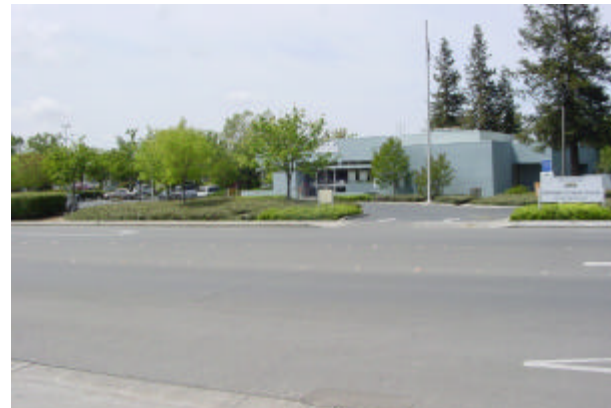
8 - Looking West at DMV office at Pole Line & 5th
