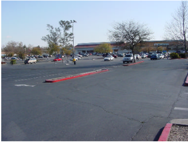
1 - Looking South across lot
