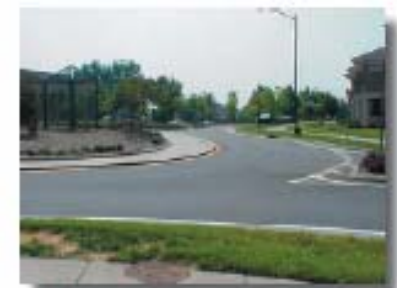
A roundabout can slow traffic without making the motorist actually stop.
