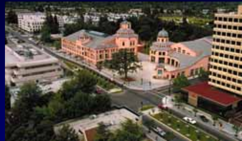
Castro Street New Civic Center After
