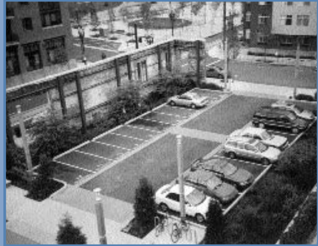
Parking lot with bio-swales in Portland, OR.
