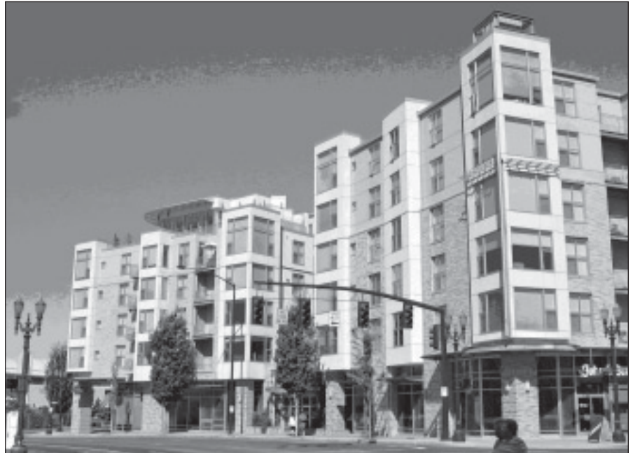
Figure 1. TOD housing produces considerably fewer trips than conventional development. The Merrick in Portland has an actual trip generation rate of 2.01 compared to the average ITE trip generation rate of 6.72 that was originally assumed for the development.
