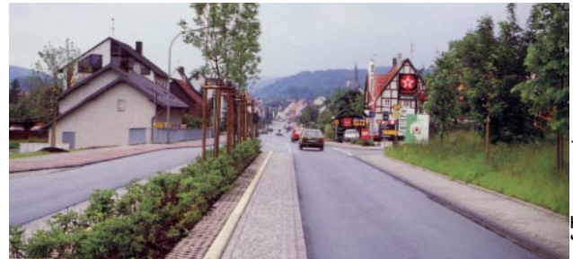
Raised and Landscaped Median
